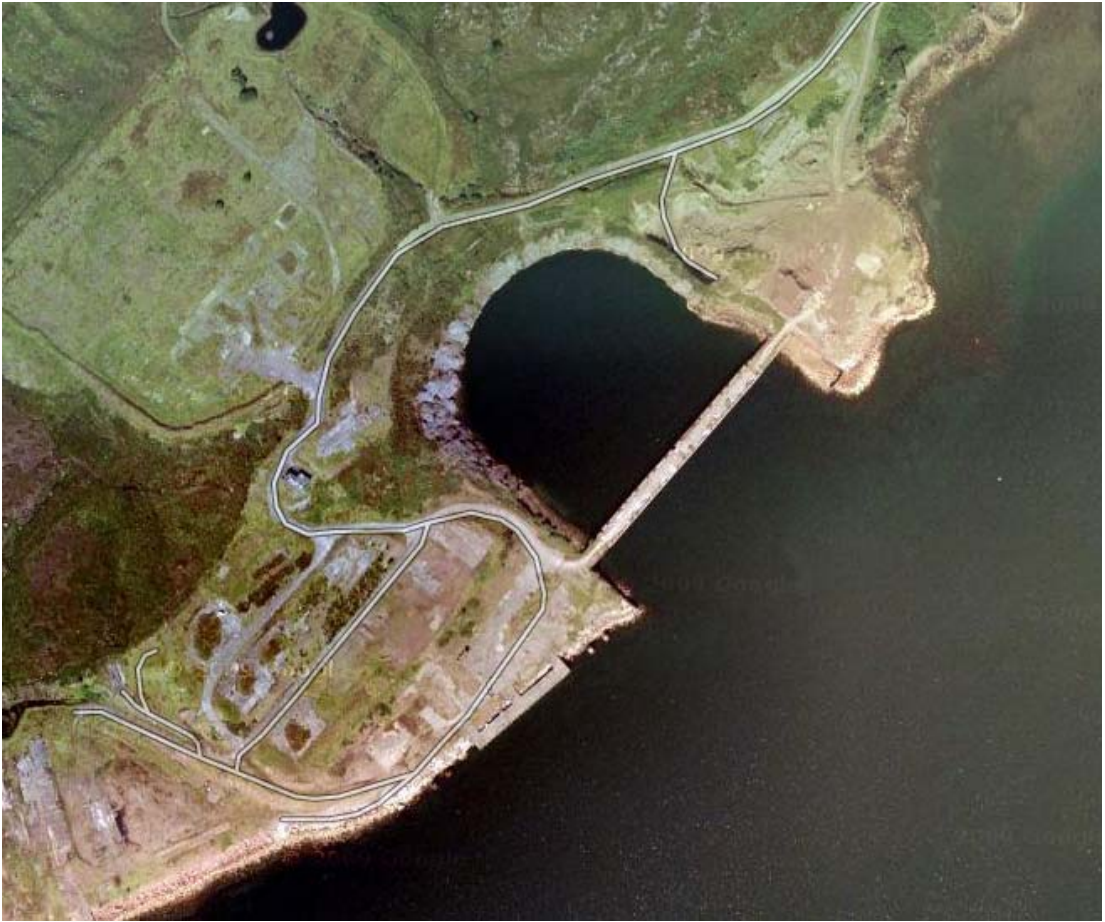
Figur 5-4: Kishorn Yard, satellittfoto
