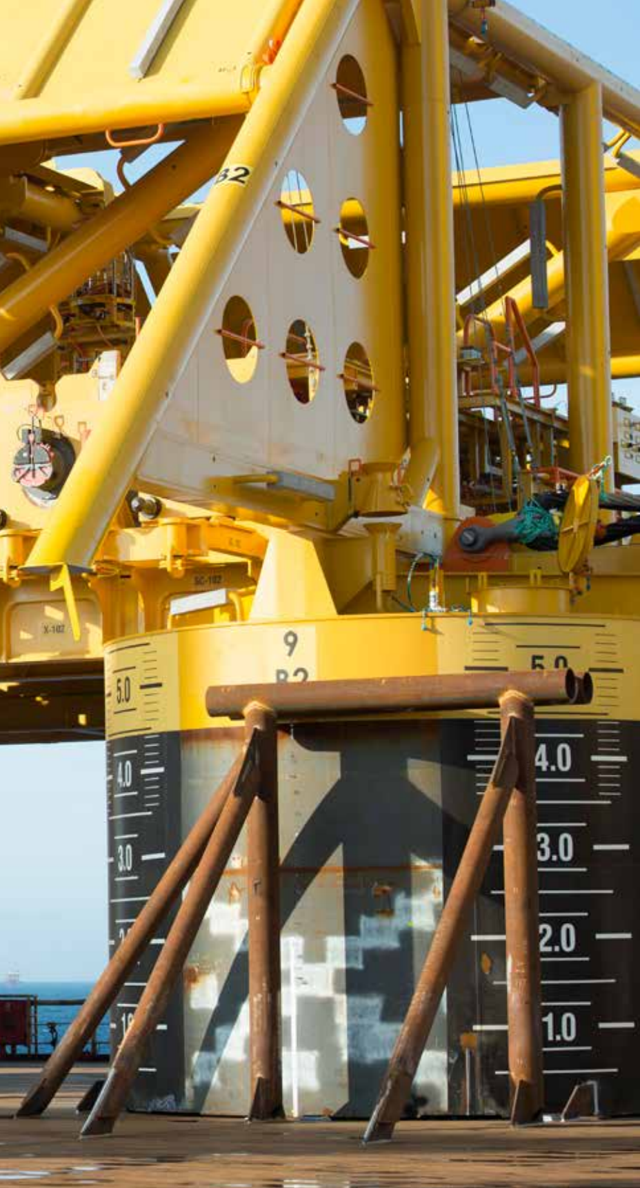
Big dimensions. The subsea compressor station on Åsgard is the size of a football pitch. (Photo: Statoil/Øyvind Hagen)
