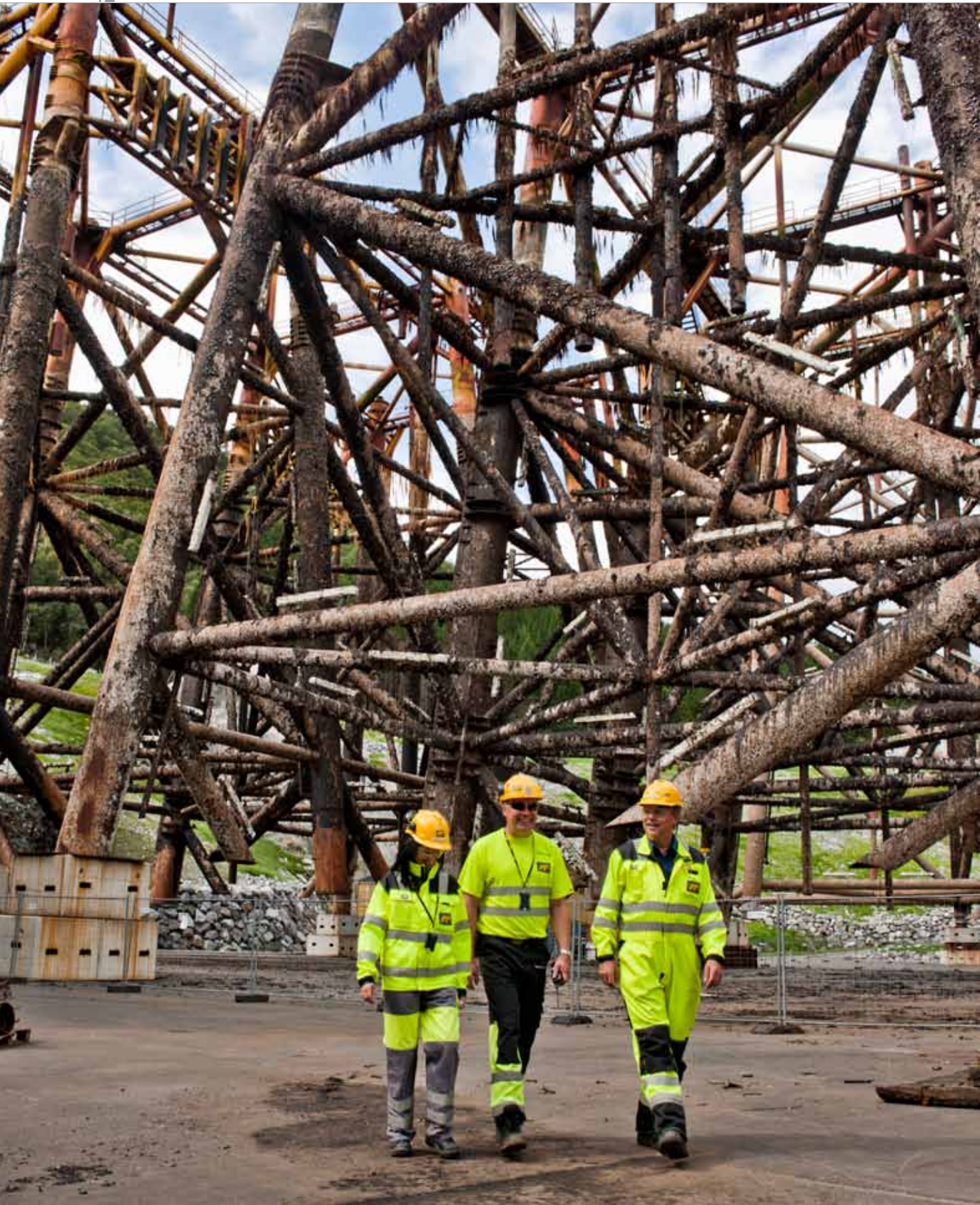
IN THE SEA FOR 35 YEARS. The closer to the sea surface these bracings have been, the more growth on them. (From left) Evy Lærdal, Bjørn Hundhammer and Arne Skogheim.
