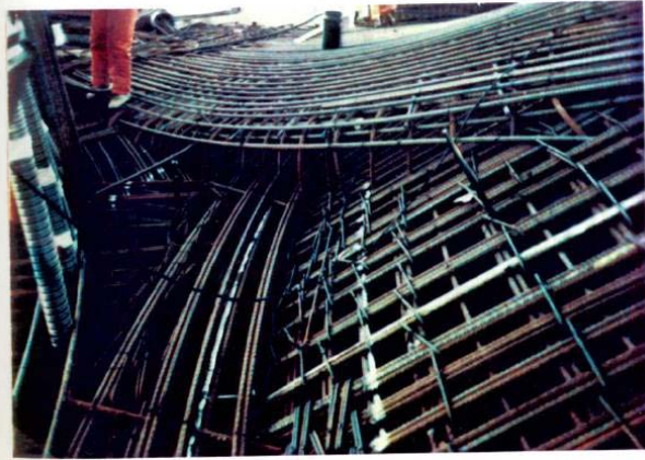
Figure 10 Reinforcement of abdominal belt [13].
