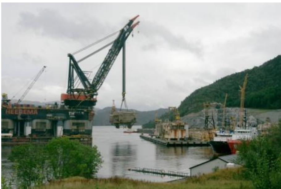
Figure 2 Heavy lifting operation: modules being delivered to the Vats decommissioning yard by a crane vessel
