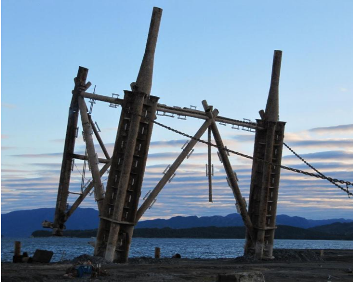
Figure 8 Steel jacket being tipped at the Aker Stord yard
