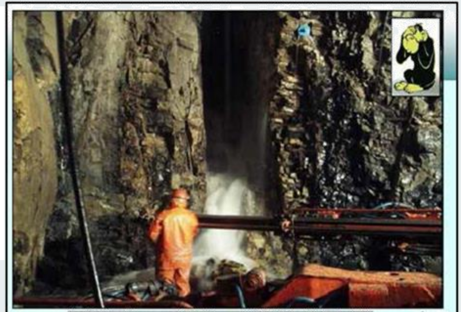
'Soil' fill collapse in an unpredicted fracture
