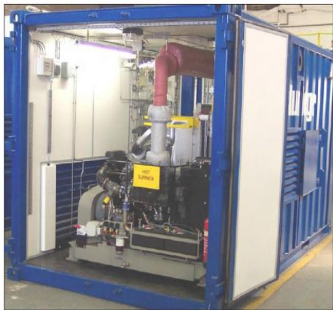
125 SCFM Compressor and/or gas quads
