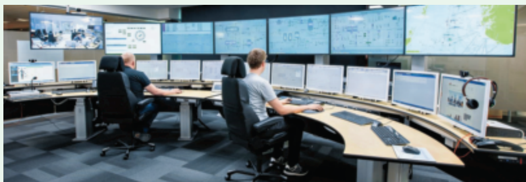
Figure 2.29 The control room for Ivar Aasen. Photo: Aker BP
