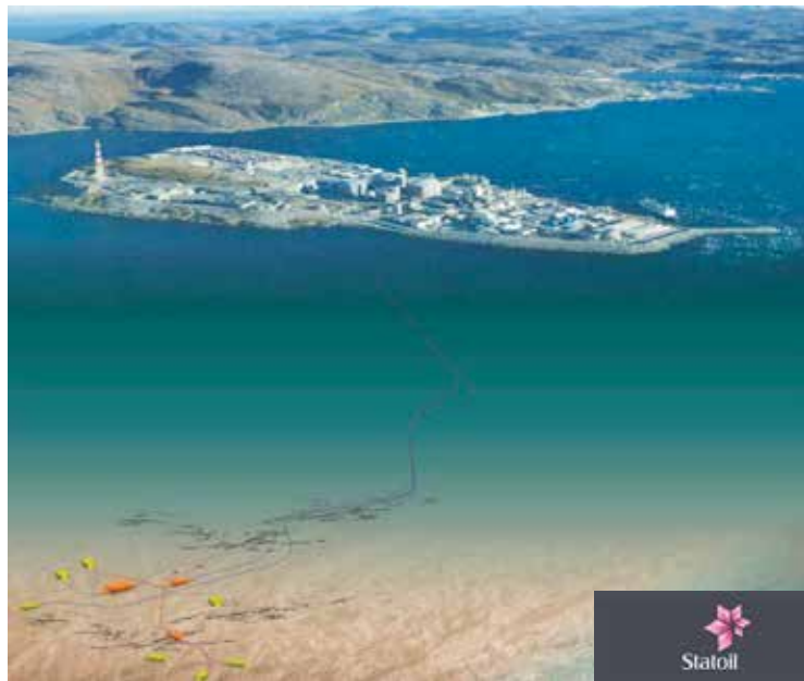
Snøhvit: There is capacity for separation and storage of 700 000 tons annually in water-saturated sandstone reservoirs under the Snøhvit Field in the Barents Sea. A shale cap which lies above the sandstone will seal the reservoir and ensure that the CO 2 stays underground.
