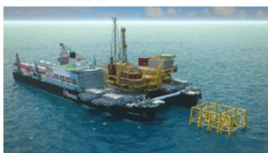
7. The vessel moves away from the jacket; the sea-fastening is locked
