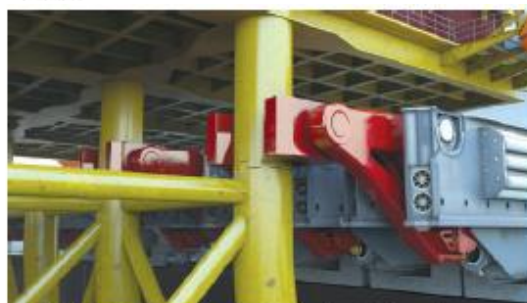
4. The horse shoes are connected to the platform legs
